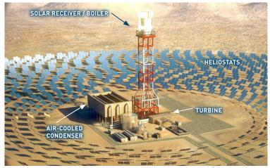
• This high-temperature steam is then piped from the boiler to a standard turbine where electricity is generated. From here,
