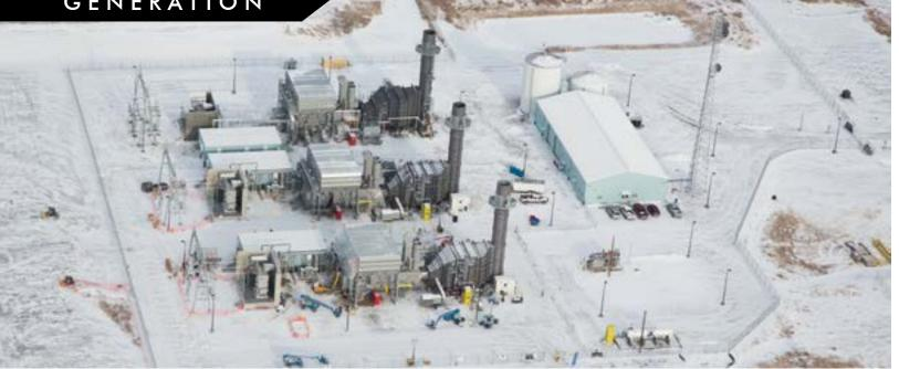
Pioneer Generation Station has three units of 45 MW of generating capacity each. Photo courtesy of Basin Electric Power Cooperative.
